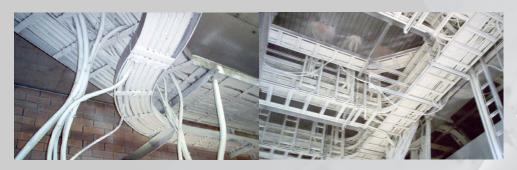
KBS Cable Coating is a water based ablative (non-intumescent) fire protective cable coating especially developed for the fire protection of grouped or bundled electrical cables and for penetration seals. Tough, flexible, water and weather resistant, it has been used worldwide since 1967 for interior and exterior applications.
